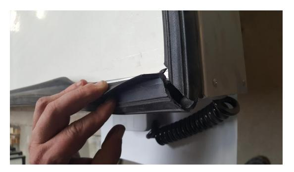
2) Disconnect heating cable from the box and remove it from gasket.
